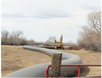
Sections of large-diameter PE 4710 HDPE pipe were fused together to make a leak-free line that runs 21 miles to provide water under pressure to irrigate some 53,000 acres of farmland in northeast Utah and saves \$50,000 annually. The undertaking was named Project of the Year for the Plastics Pipe Institute's Municipal and Industrial Division.
